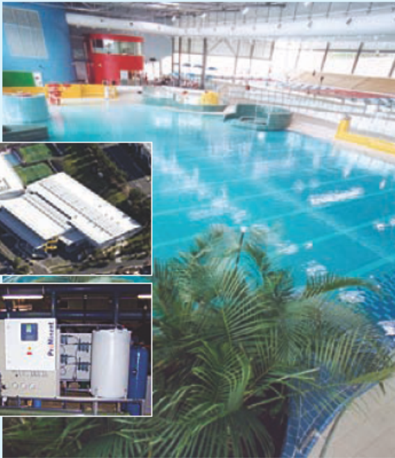
Ryde Aquatic Leisure Centre with Backwash Recovery System
